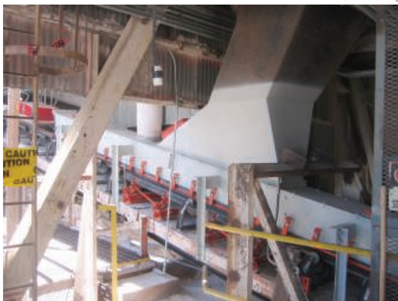
FIGURE 3. Dust containment can be improved by enclosing the settling zone to slow the air velocity and return dust to the cargo flow
