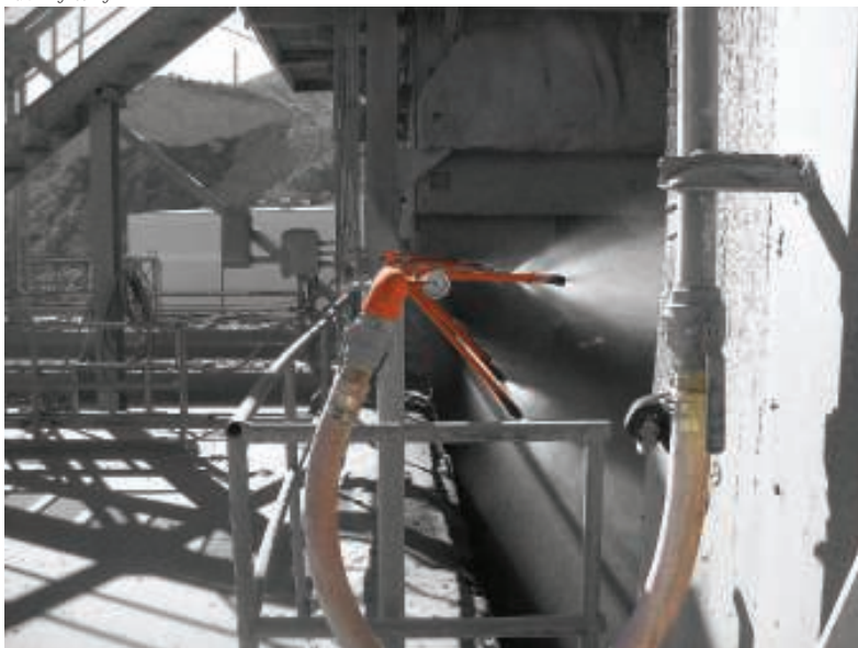
FIGURE 9. Dust suppression involves preventing dust particles from leaving the material stream
